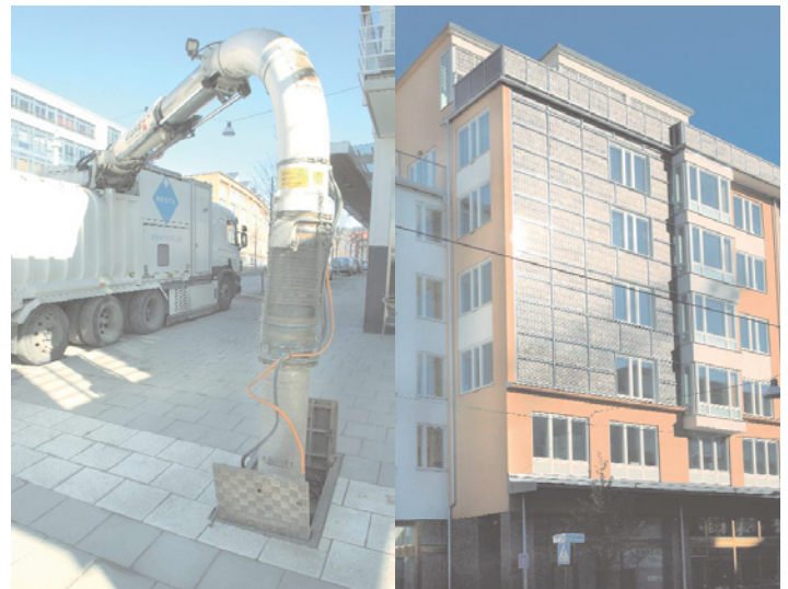
Vacuum Trash Pickup / PV Array Built into Facade
