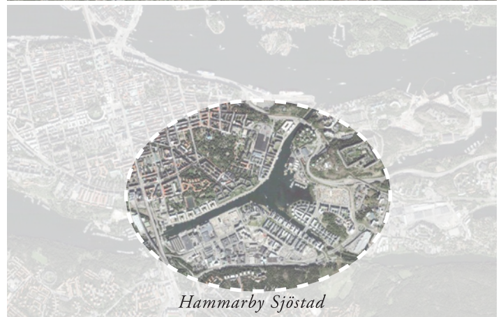
Aerial Site Photos
